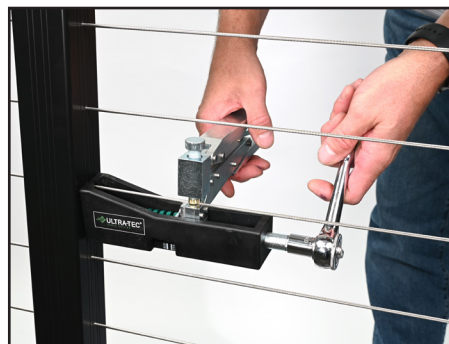
Rotate using ratchet to pull tension
