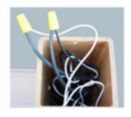
Cut and snip fixture wires and main wires to comfortable working length.
