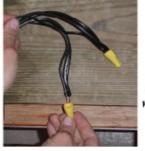
RECESSED 6 Cut and snip fixture wire and (2) main wires to comfortable working length and connect with a UL approved silicone wire nut. Be sure at least 7/16" of copper wire is exposed and wire nuts are on securely. Loose connectors can arch causing fixture failure or fire.
