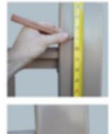
Determine where the fixture is to be installed and make a reference mark for centering the mounting and wire hole. Tip: measure from the top of the deck to the desired top of light height (usually around 34") and make a mark. Next, measure from left to right across the post and divide this # in half and mark. Center is where the two marks intersect.
