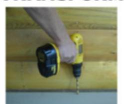
Drill a 3/8" hole through the deck surface and feed main line through to the under side of deck. Next, run the main wire to your first fixture. Secure the main wire using insulated staples or cable tacks. Tip: For faster installation pre-wire the main run before decking is installed!
