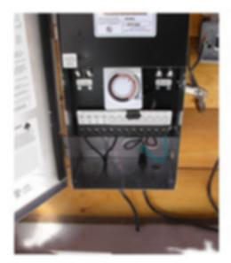
Using installation instructions provided with transformer, mount transformer to house and install main power feed line. This line should be a UV resistant, UL approved 12-2 low voltage cable with a 100' max run and no more than 250 watts. If run is more than 100' and over 250 watts, use 10-2 or 8-2 wire to carry the load. Be sure main line is long enough to reach the first lighting fixture.
