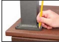
Mark and Pre-drill Holes
