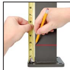
Measure up 2-1/2" from top of base plate
