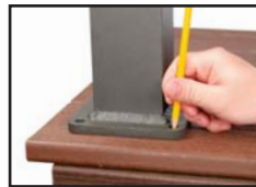
Mark and Pre-drill Holes
