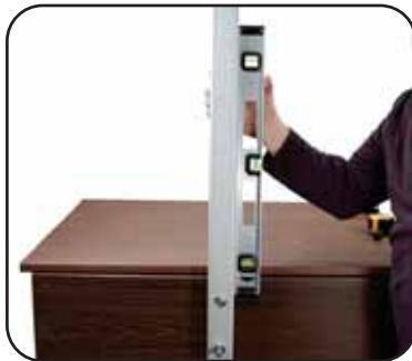
Step 10: Plumb post, adjust as needed. Tighten fasteners and ensure proper engagement into blocking.
