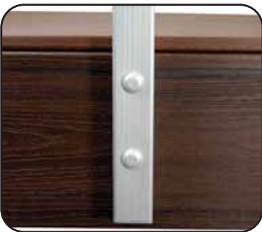
Step 12: Finished fascia mount post installed.
