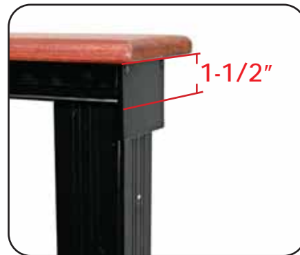
(2) Mark Reference Line Measure down 1-1/2" from the top of the extended end plate and mark a temporary line. (Keep end plate tight to post)
