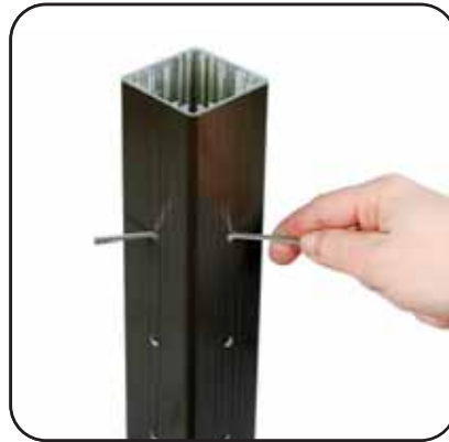
Step 2: Insert Cable Insert the cable into each hole and pass through the post. Make sure not to fray the end of the cable while feeding through the post.
