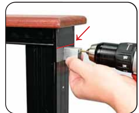
(3) Locate Rail Connecting Block (RCB) Align the RCB with the line made in Step 2 and center the RCB on the extended end plate. Pre-drill the end plate with 5/32" drill bit using the RCB as a guide.
