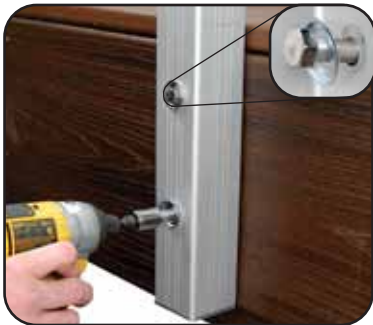
Step 9: Install cup washer under head of each fastener and drive fastener loosely into blocking.
