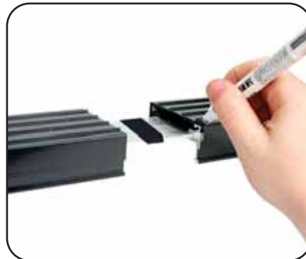
Painting Top Rail Ends (Optional) It is recommended to paint the rail ends / splices for an inconspicuous splice seam. Also prevents oxidation. Applies to all colors.
