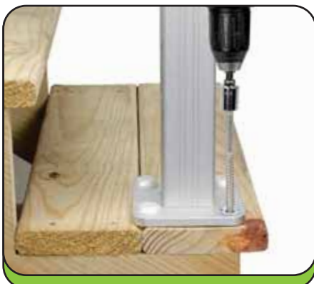
Step 16: Attach post to surface.
