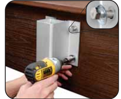
Step 2: Attach bracket to fascia
