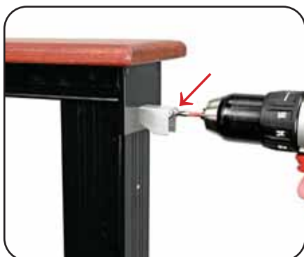
(5) Attach RCB to End Plate Attach the RCB to the extended end plate. Attaches with 2 ea. screws using #2 square drive.
