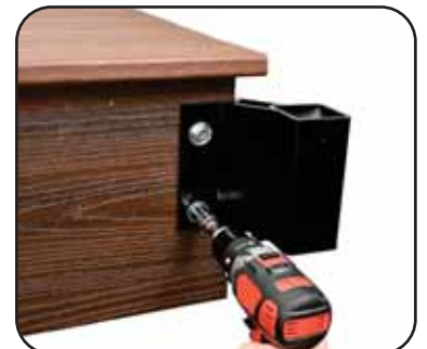
Step 2: Attach bracket to fascia
