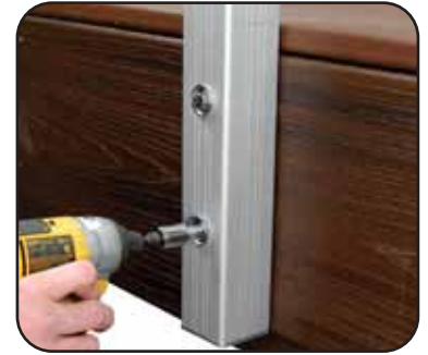
Step 8: Determine location of fascia post. (Max. post spacing of 60" on center) Mark holes, remove post and drill pilot holes to accept 3/8" lag or carriage bolt.
