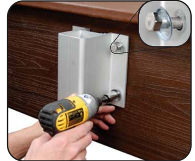
Step 2: Attach bracket to fascia
