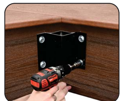
Step 2: Attach bracket to fascia
