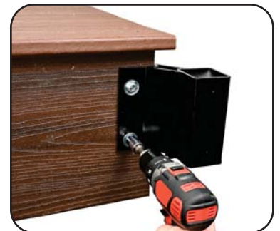
Step 2: Attach bracket to fascia
