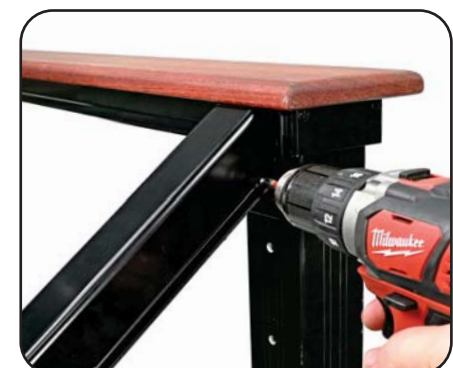
(9) Attach Top Rail Attach top rail to RCB using 1 screw on each side. Screws should be offset slightly to avoid colliding inside the rail.
