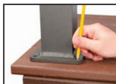
Mark and Pre-drill Holes
