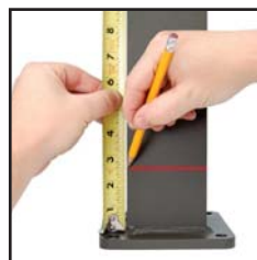
Measure up 2-1/2" from top of base plate
