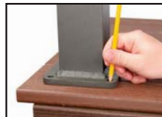
Mark and Pre-drill Holes
