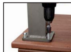
Fasten Post to Deck Surface
