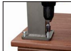
Fasten Post to Deck Surface
