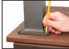
Mark and Pre-drill Holes
